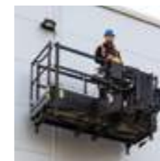
Man platform ready
